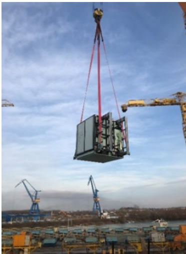
Transport of Climeon's modules on the way to installation
