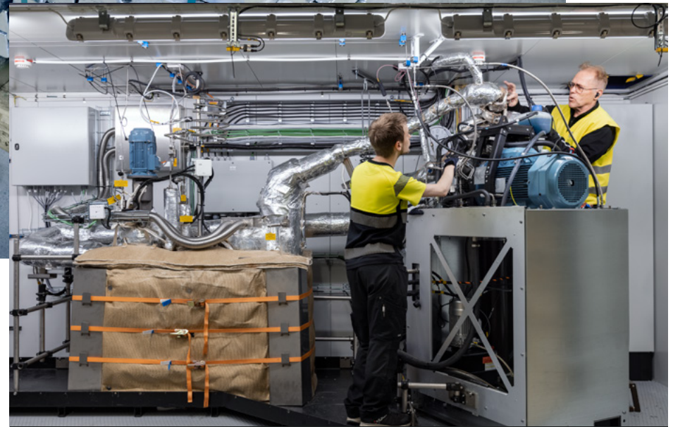
Energy is stored in long-duration energy storage units of recycled aluminium, a material whose storage capacity does not degrade over time.
