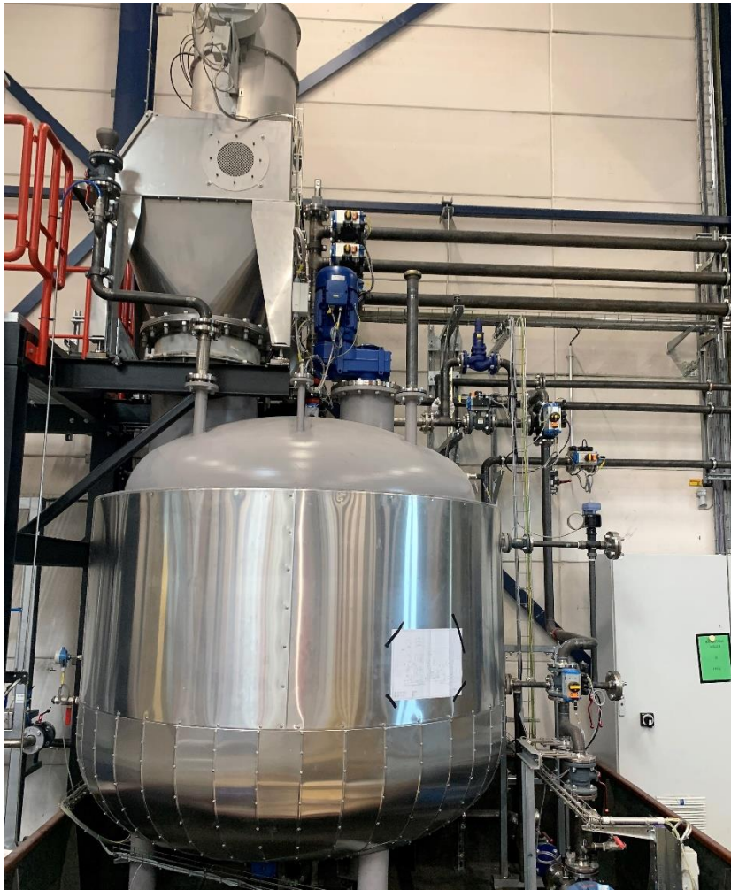
Equipment for incorporation of Quartzene® at a customer's production facility.
