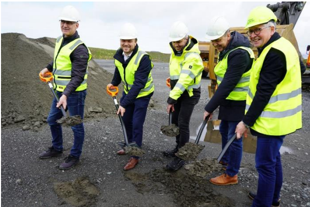
Construction start ceremony
