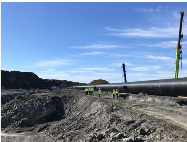
Wastewater pipe before putted into ground
