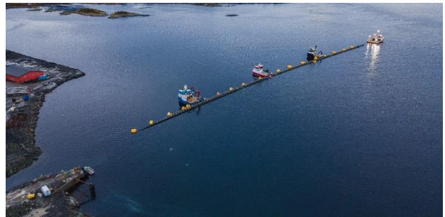
Installation of water inlet pipes (October 2021)
