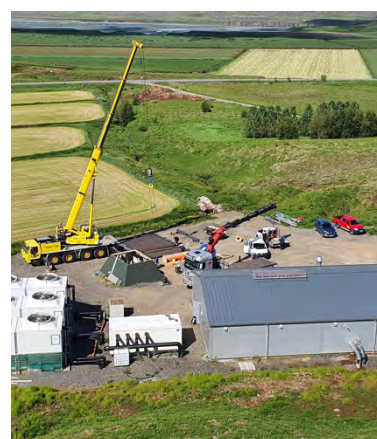
The Climeon modules in Varmaorka's power plant in Fludir had an availability of 98.3 percent in 2020, well above the target.
